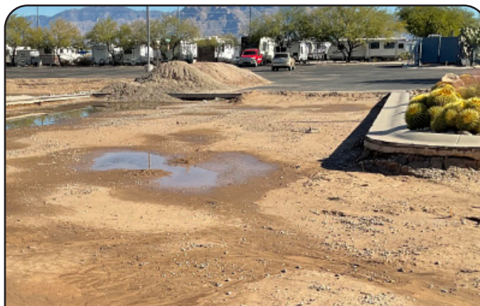
Saturated subgrade in driveway, remove and replace where necessary.
