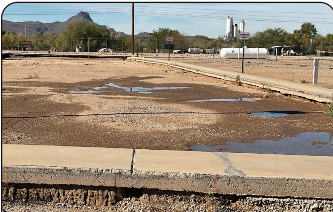
Center of driveway drainage swale. Confirm all elevations- remove and replace where necessary.
