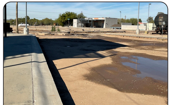
Rolled curb at sidewalk. Confirm that all subgrade beneath acceptable. Remove & replace where necessary.
