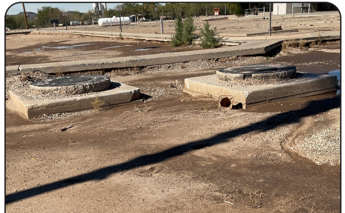
Electrical and Communications manholes. Confirm all elevations and reset if necessary.
